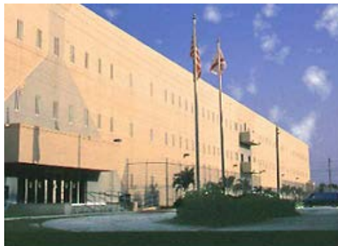
3,098-Bed Metro West Detention Center, Miami, FL
