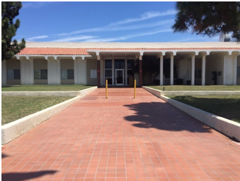
SANTA BARBARA COUNTY JAIL VISITOR'S ENTRANCE
