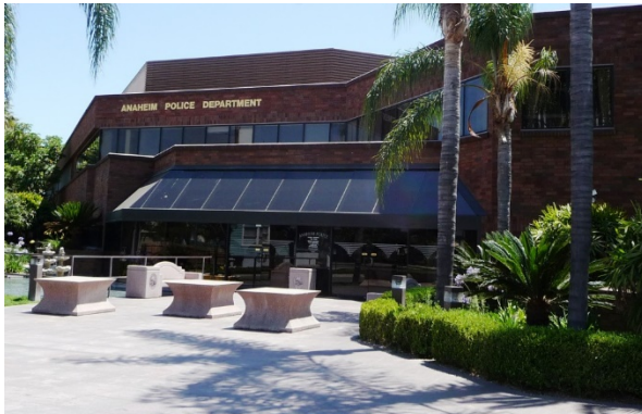
ANAHEIM POLICE DEPARTMENT, WHERE THE DETENTION FACILITY IS LOCATED.
