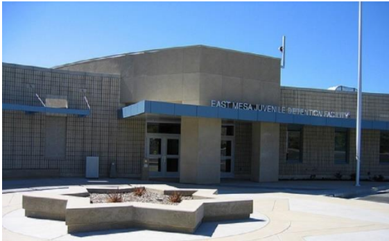
East Mesa Juvenile Detention Facility, San Diego, CA
