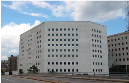
Monroe Co. Public safety Building (Rochester, NY)
