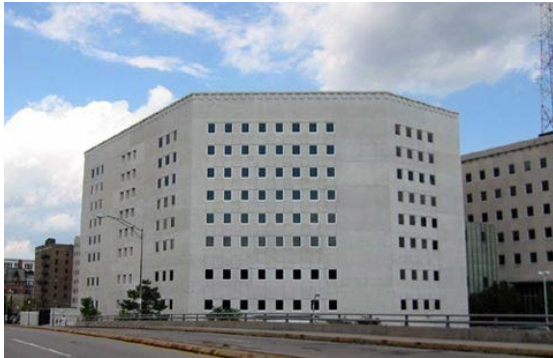
MONROE COUNTY JAIL. (PHOTO: MONROECOUNTY.GOV)
